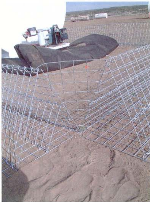
Triangular basket panels have an interior strut for strength and reinforcement.
